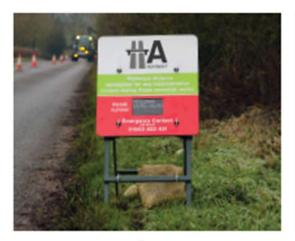
Intelliframe® is an innovative way of digitally monitoring and managing street works to ensure compliance with relevant legislation, provide real-time updates to road users and allow remote visibility and monitoring of physical diversions.
