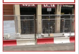
Heavv duty traffic/pedestrian segregation barrier that self-stabilises when and errant vehicle hits the system. Can be fitted with a variety of top units.
